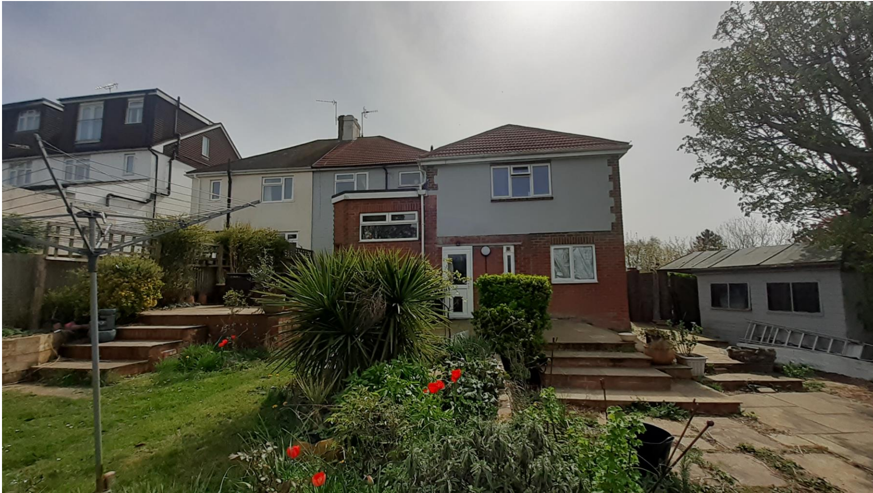
Existing rear garden at 65 Ladies Mile Road
